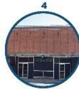
4 108 Montcalm St. Building Rehabilitation
